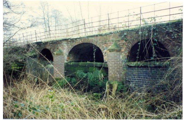
A photograph of the bridge taken about 20 years ago
